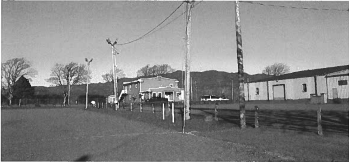
Overhead lines to be removed on West side
