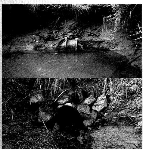
Description: Bandy Slough is a small slough on the North Fork Nehalem. A tide gate and berm disconnect the historic wetland and flood plain from the river. Three private landowners have agreed to remove the tide gate. The removal will need to accommodate an easement for accessing power lines on site.
