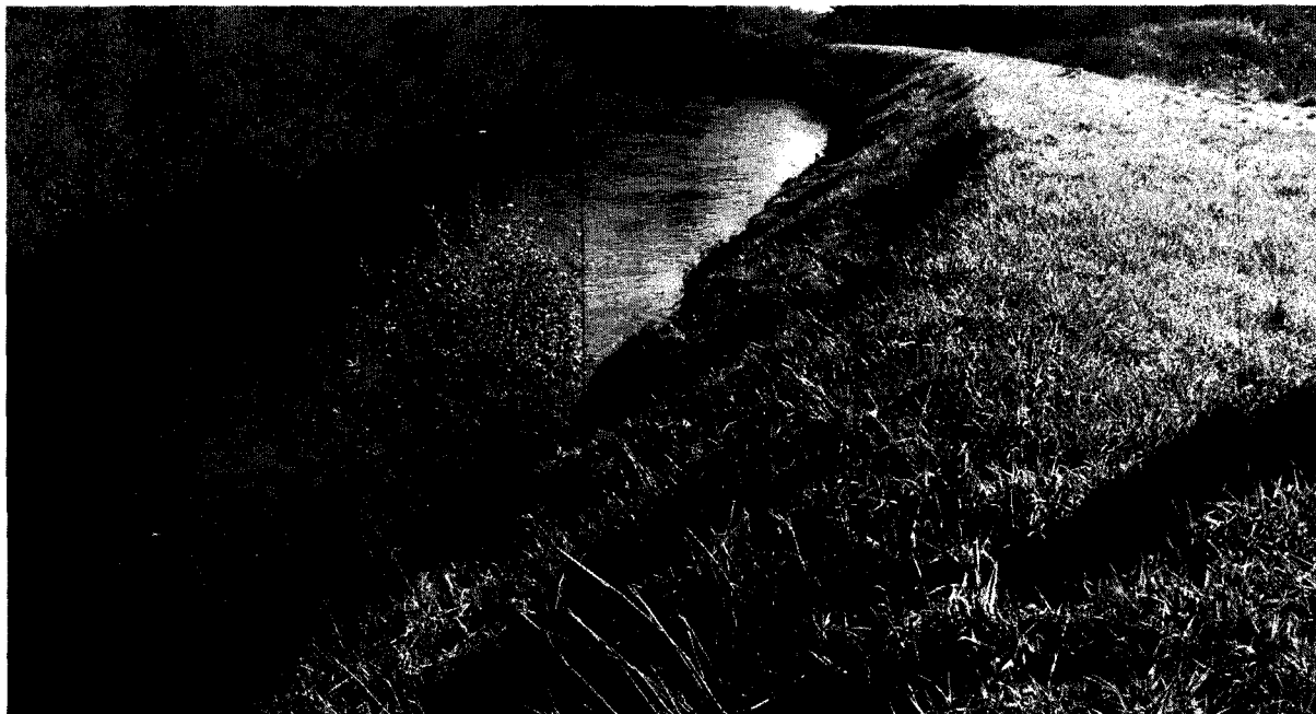
Middle and upper portion of revetment looking upstream. Note small willow needing to be cut.
