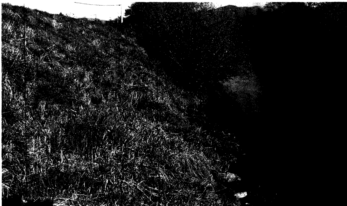
View downstream from near Sta. 8+00. Some riprap exposed at waterline. Trees need to be removed from slope or at least have back sides cut to reduce drag during high water events.
