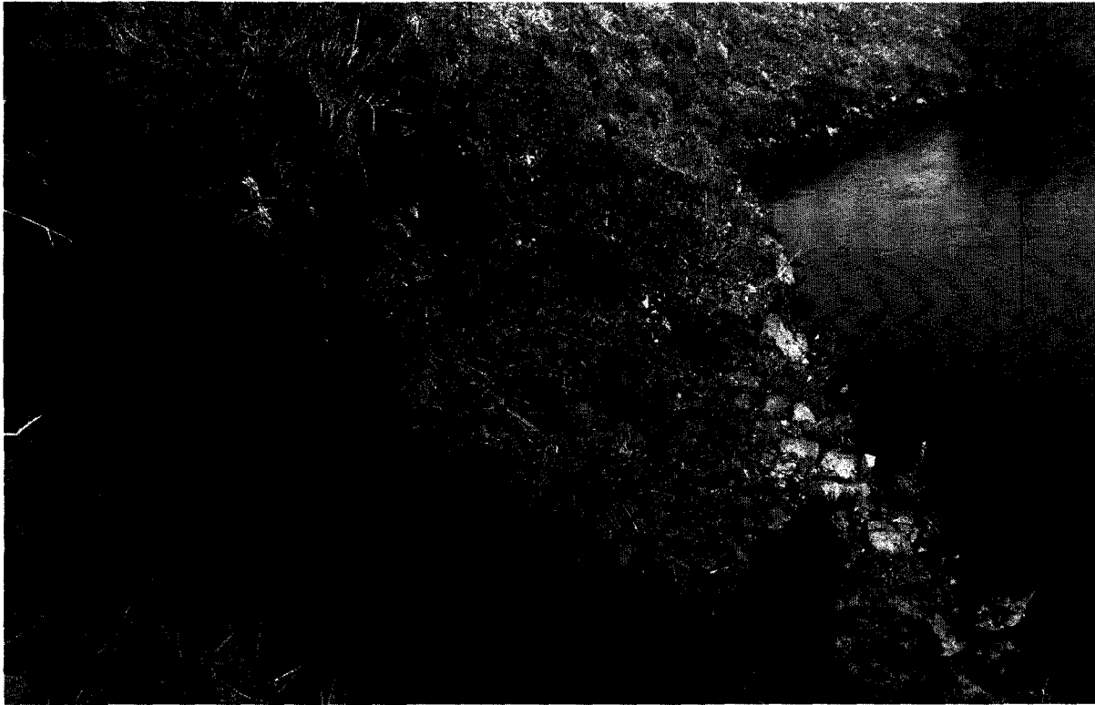
Close-up of area just before bend where river has eroded the overlying thick silt layer present on the 1V:2H riprap slope. Any lost riprap needs to be replaced to restore slope integrity.
