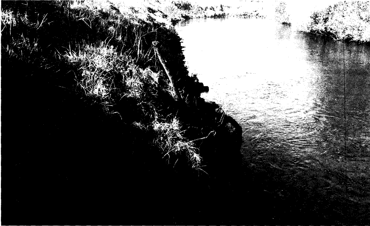
Woody debris caught between slumped blocks of silt on lower slope of revetment. Should be removed to prevent additional debris from getting caught and exacerbating erosion.
