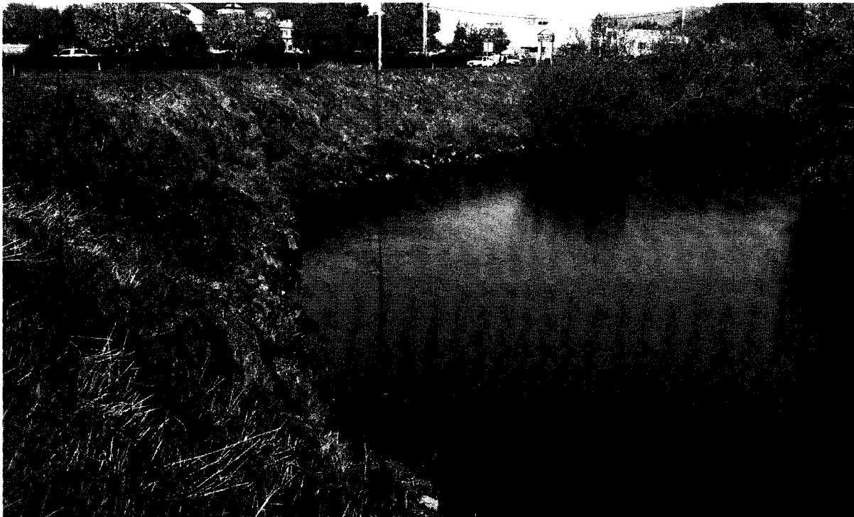
View D/S of overlying silt erosion on lower slope exposing riprap between Sta. 7+00 to 8+00.
