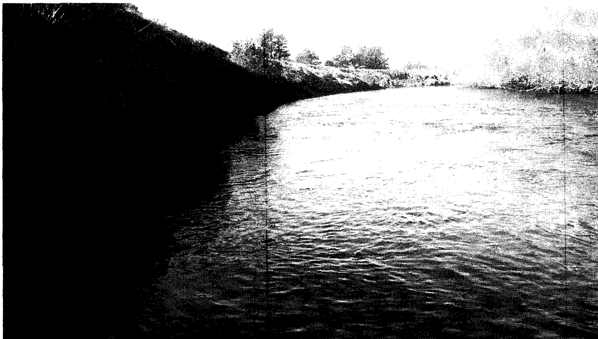
View downstream of riprap exposed at waterline taken from U/S end of revetment. Note the thick layer of silt creating an oversteepened slope that is overlying the 1V:2H riprap slope.
