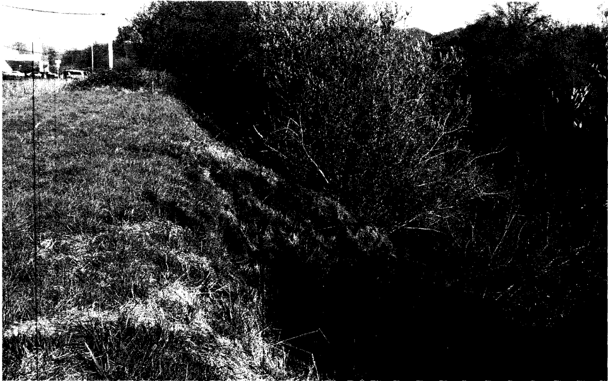
Areas of large willows growing through lower end of revetment slope. Numerous slumped silt areas present in this area. D/S end of project is located just beyond the blackberries on crest.
