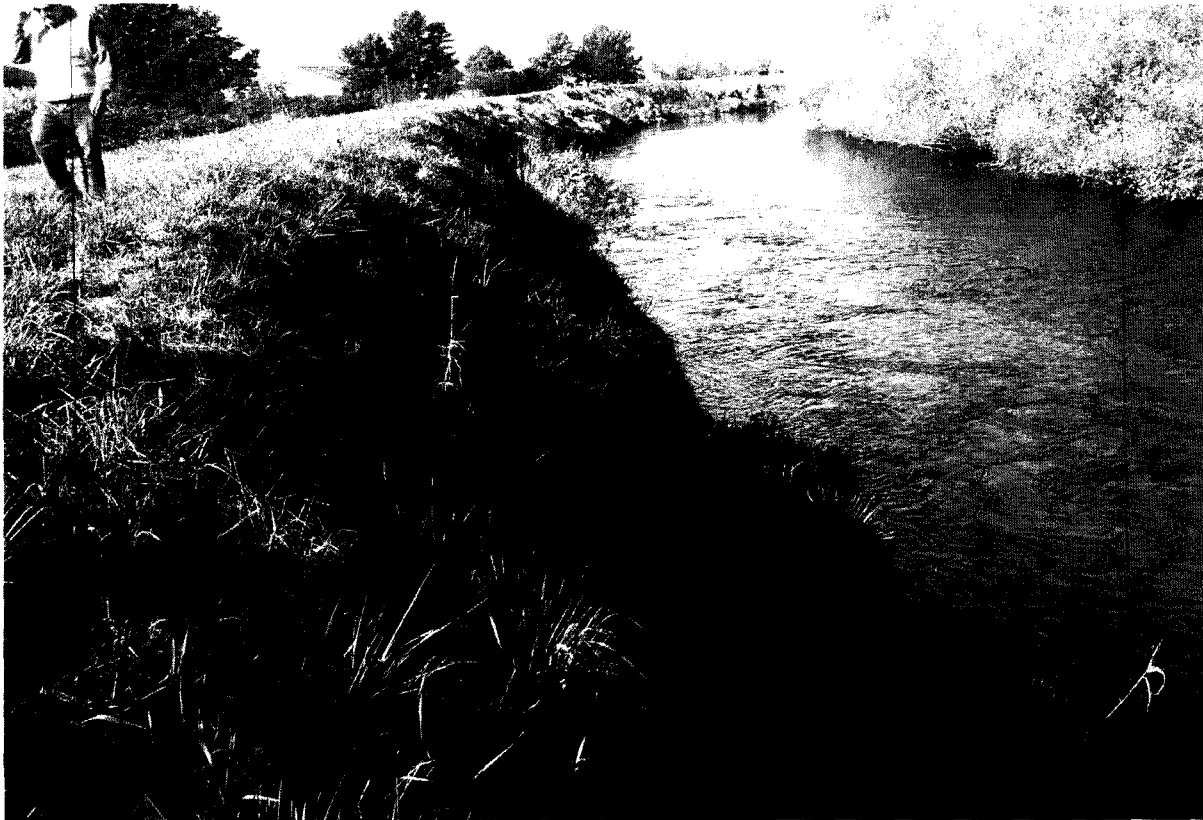
View downstream from upstream end of revetment. Riprap not visible from top of slope.
