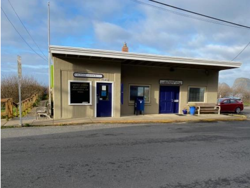
Oceanside Community Club roof repair $55,000
