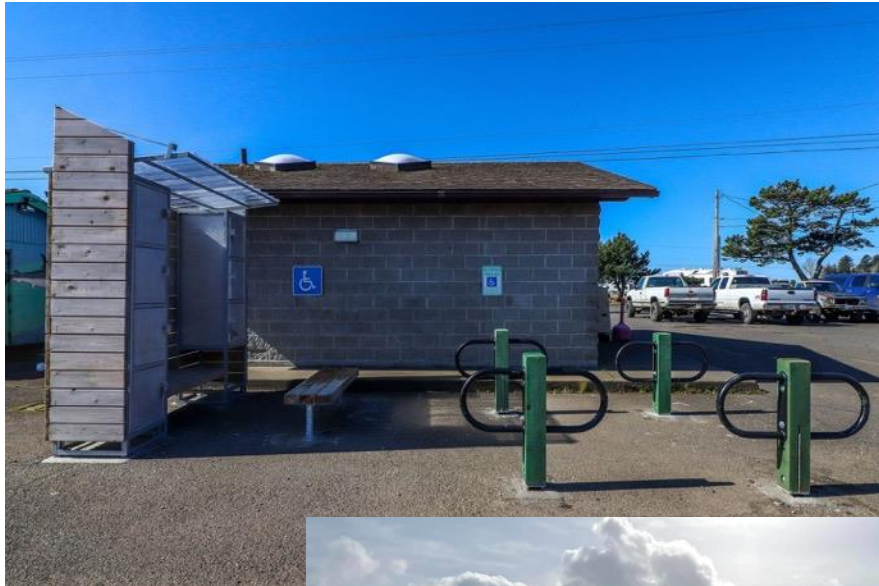
Restrooms and kiosk
