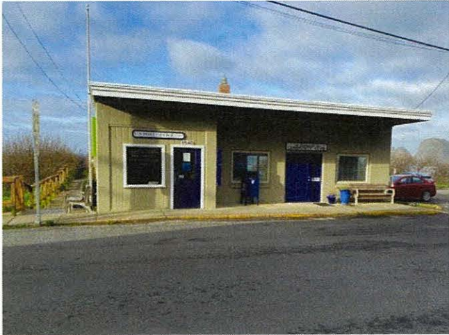
Oceanside Community Club roof and parking lot repair $113,000
