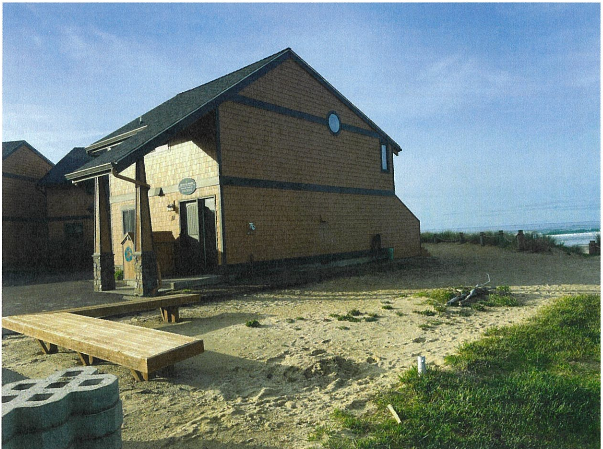
The lot has been cleared and cleaned up post fire. It is ready for us to rebuild on it.
