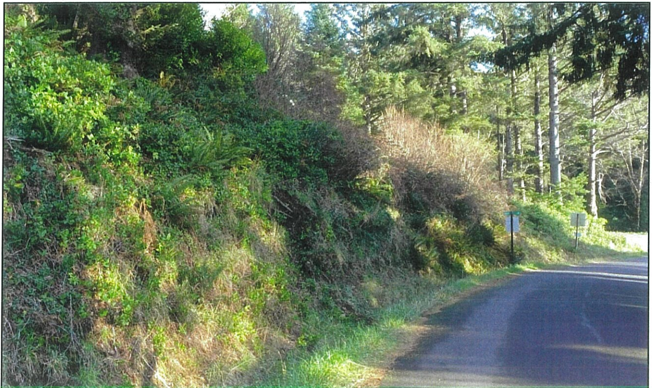
Photograph 2- View to southwest on Chinook Avenue, steeply sloped Tax Lot 700 and Chinook Avenue right of way at left in photograph.
