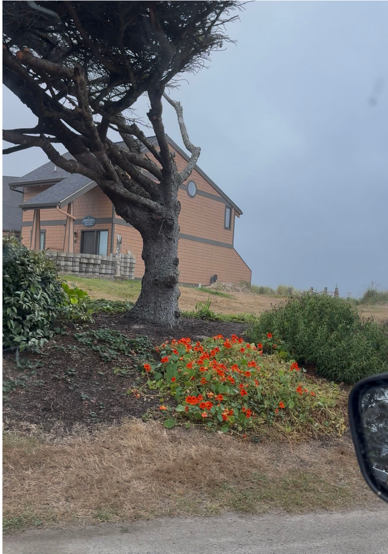
GRADE DIFFERENCE AT BREAKERS CONDOMINIUM
