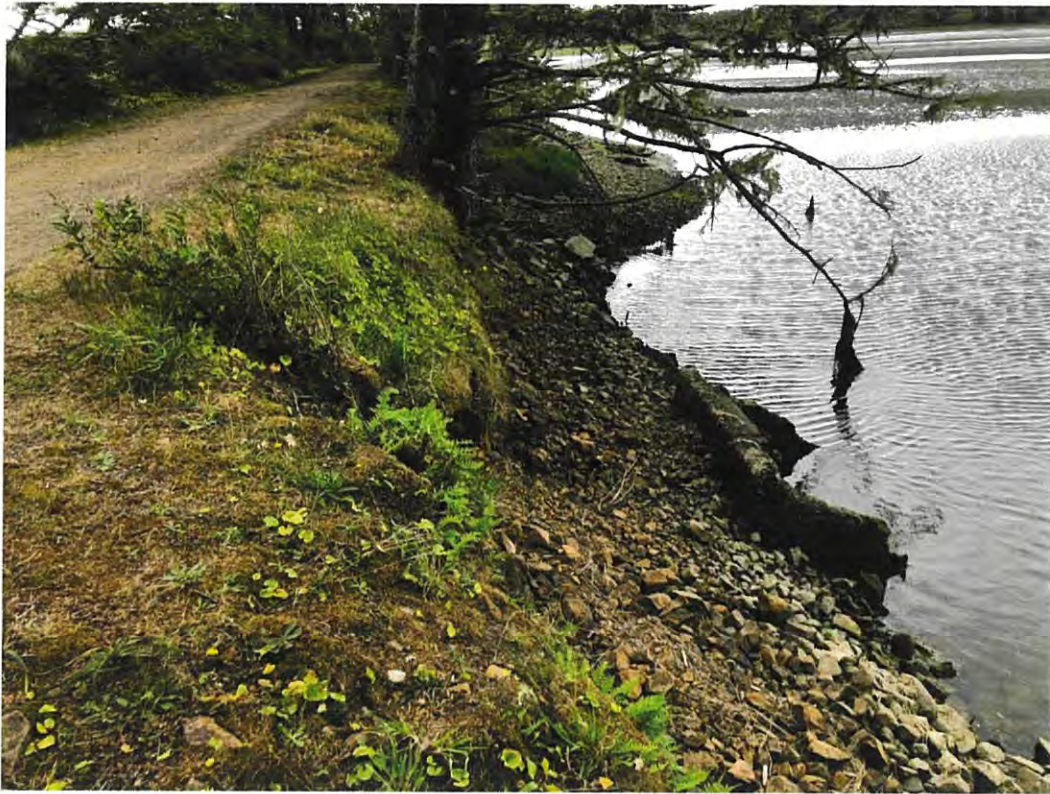
Exhibit 7-1: View east, at the existing tidal gate within Beltz Dike.
