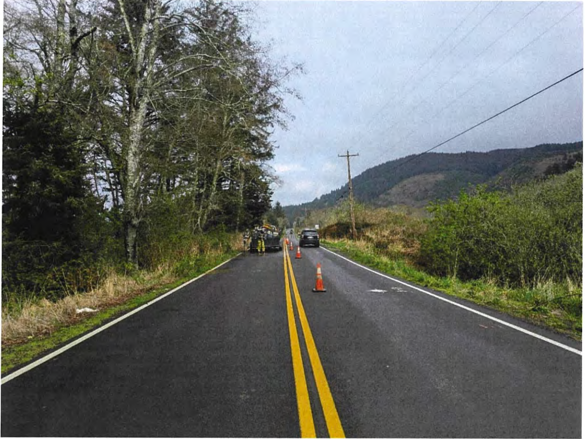
Exhibit 2-6: View northeast along Sandlake Road within the area of Beltz Creek and the proposed bridge.
