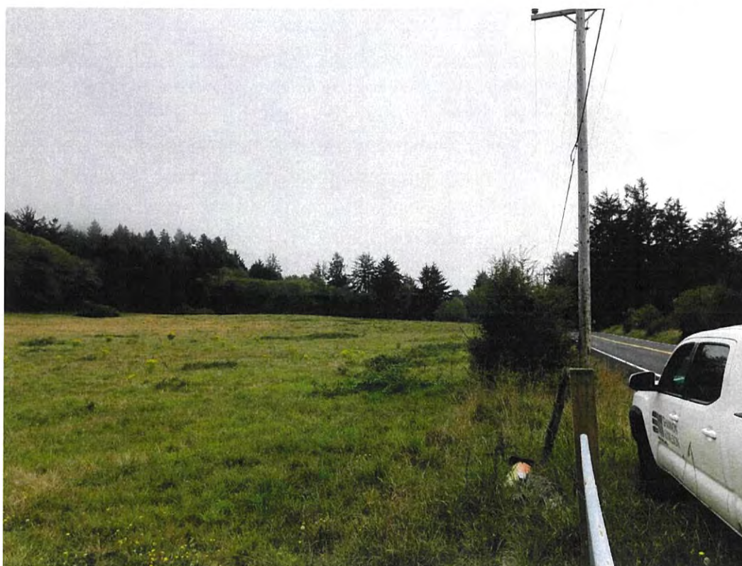
Exhibit 7-4: View southwest at the debris flow as it exits west out of the stream valley of Beltz Creek.
