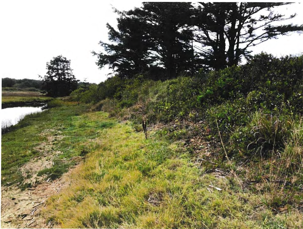
Exhibit 2-4: View west showing the slope of the embankment of Beltz Dike.
