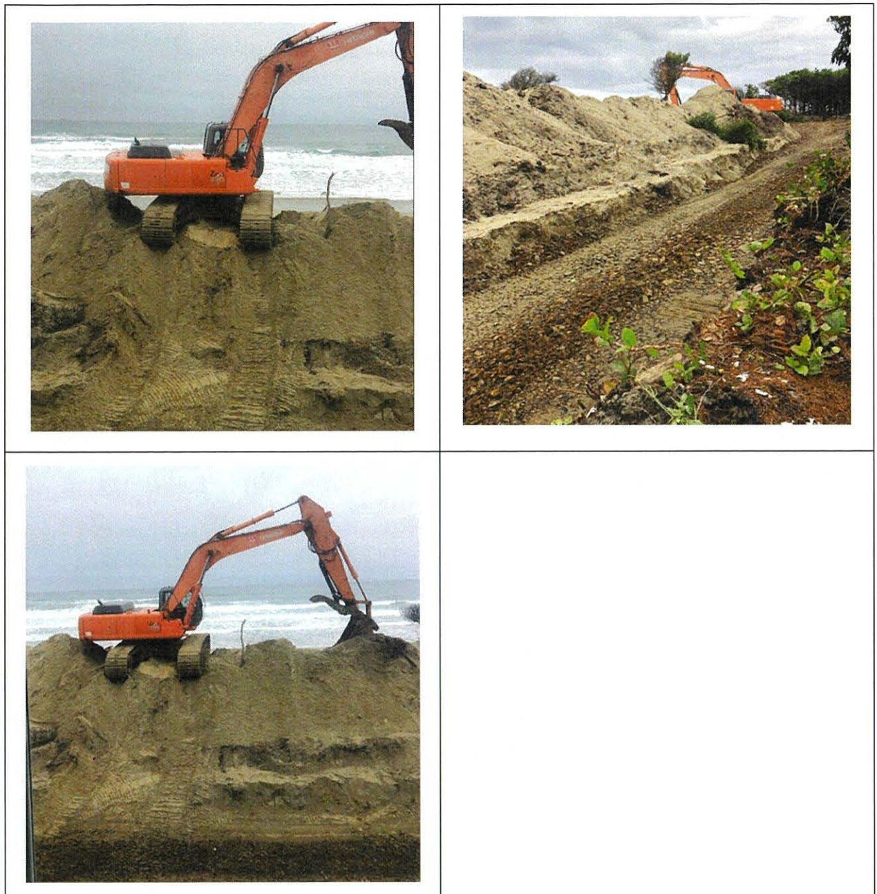
Figure 4. Photos of construction of shoreline protection revetment
