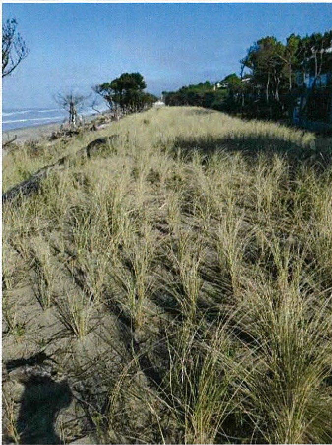
Facing North along revetment.
