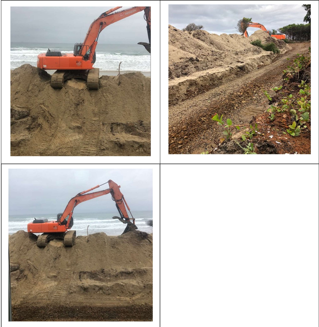
Figure 4. Photos of construction of shoreline protection revetment
