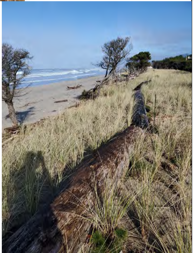
Facing Northwest showing revetment slope
