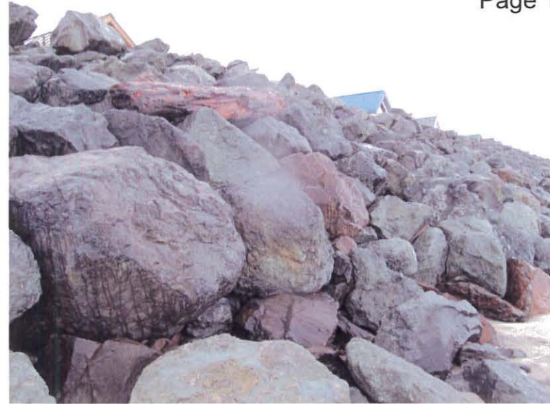
Photo 2. Close-up of rock revetment at the Shoreline RV Park located about 900 feet north of the Pine Beach subdivision.
