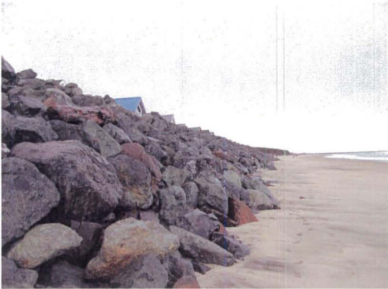
Photo 1. Looking south at the rock revetment at the Shoreline RV Park located about 900 feet north of the Pine Beach subdivision.
