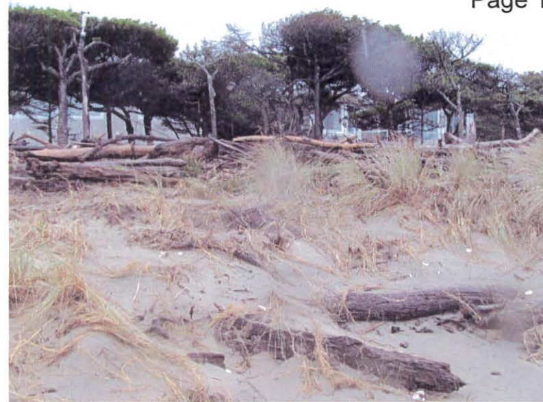
Photo 6. Looking east at the debris existing in front of the southern-most house in the Pine Beach subdivision. Note presence of large debris.
