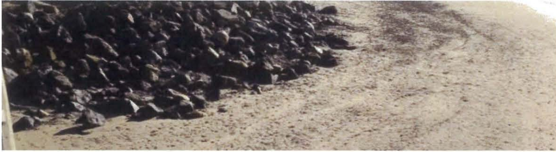
Riprap at Torrey Pines State Beach
