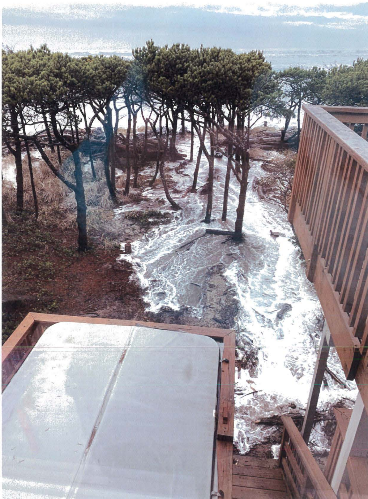
Photos of January 2021 Flooding
