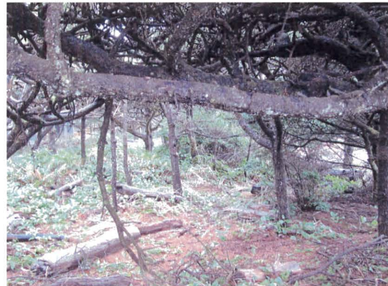
Photo 32. Looking south at the backshore bench from 50 ft south of the revetment at the Shoreline RV Park.
