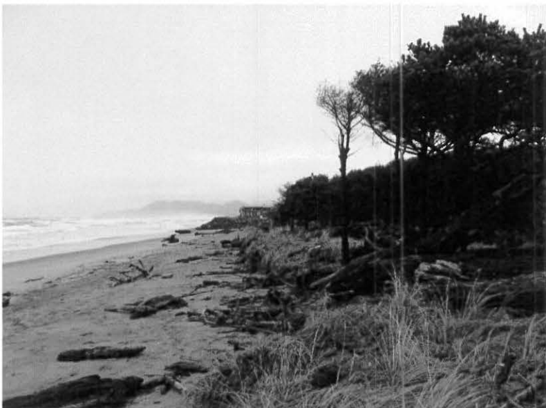
Photo 27. Looking north at the top of the vegetation line from about 200 ft north of the southern end of the Pine Beach subdivision.
