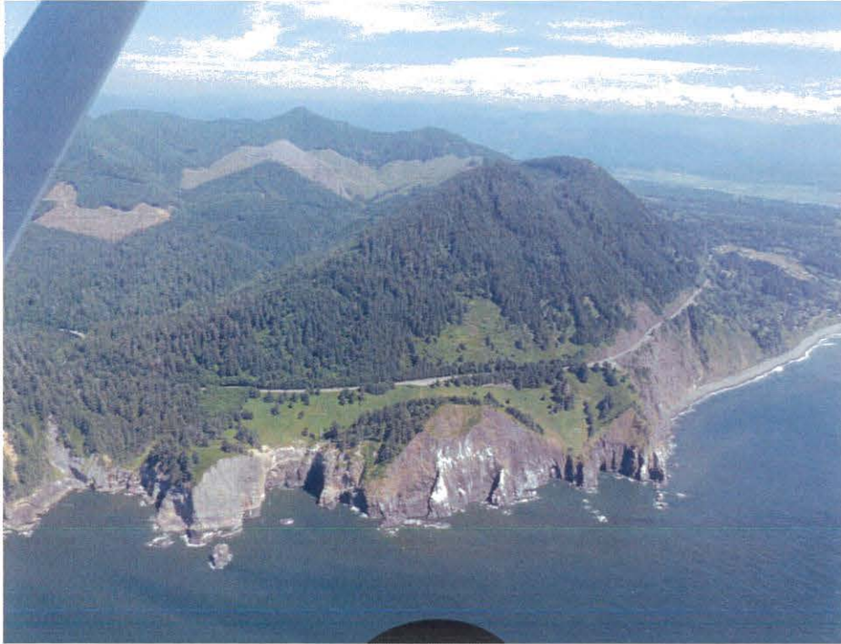
Figure 2-2. Looking east at Neahkahnie Mountain. U.S. Highway 101 can be seen around mid photo tracking along the mountain. To the right and along the toe of the bluff is an extensive cobble/boulder berm that has formed as a result of rockfalls and landslides off the headland (photo: L. Stimely, DOGAMI, 2011).
