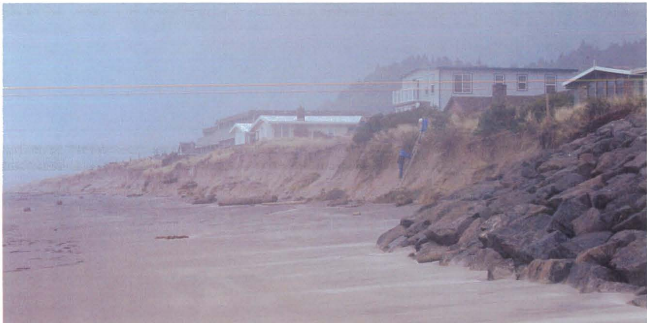
Figure 10. Dune erosion scarp that formed at Rck7 in January 2008. Note the two people having to use a ladder to get off the beach.
