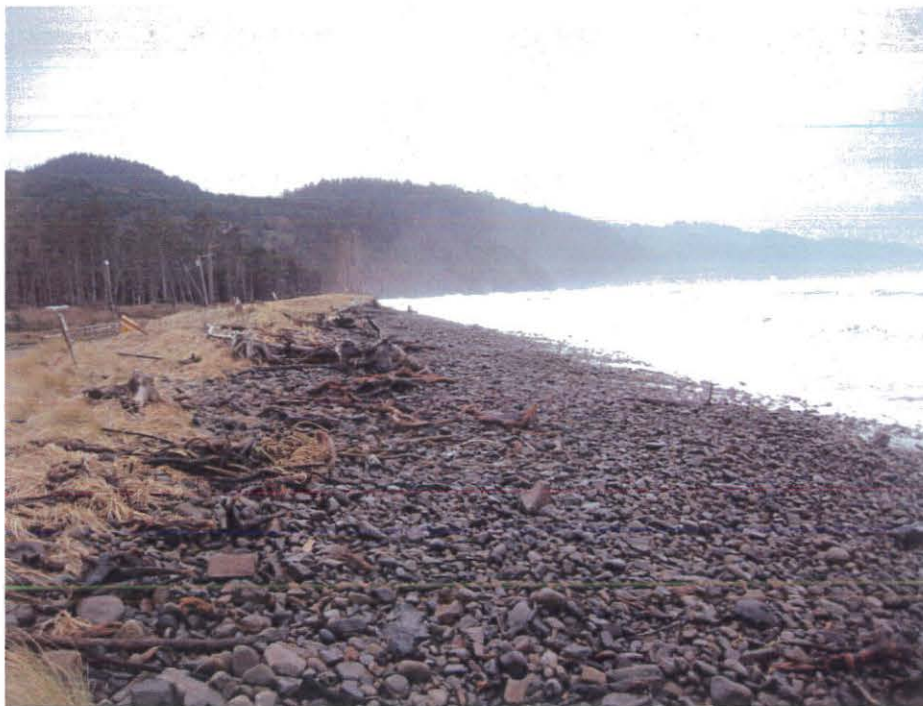
Figure 2-23. Dynamic revetment “cobble beach” constructed at Cape Lookout State Park. The cobble beach is backed by an artificial dune, which periodically is overtopped during major storms (photo: J. Allan, DOGAMI, 2008).
