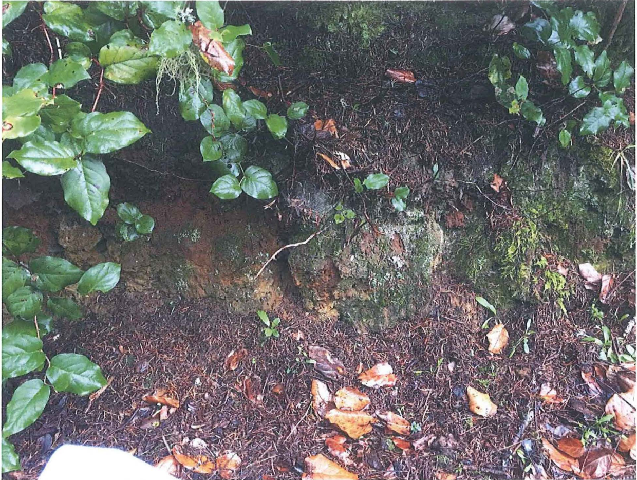
Image 3: Iron cemented sand was observed in some places. This photo was taken facing west near the top of the steep slope in the eastern part of the site.
