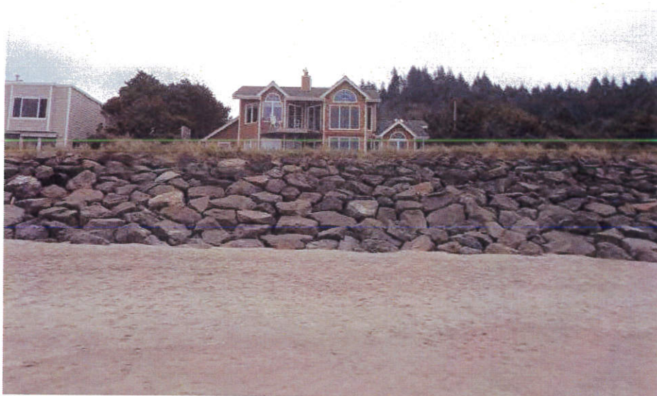
Photo 4 – Easterly view of the site and existing revetment.
