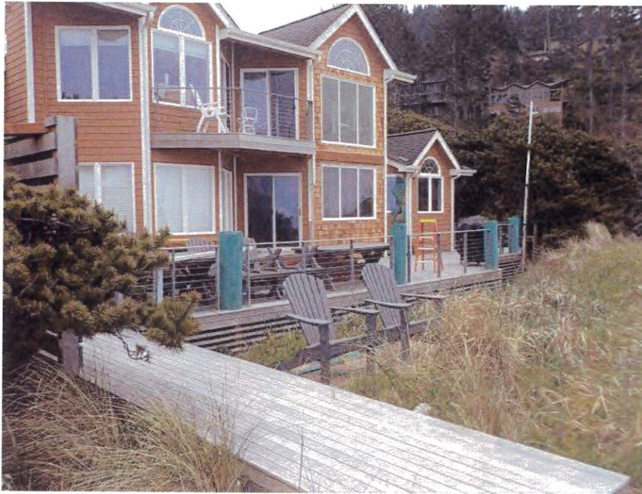
Photo 3 – View of the western side of the existing home and deck.
