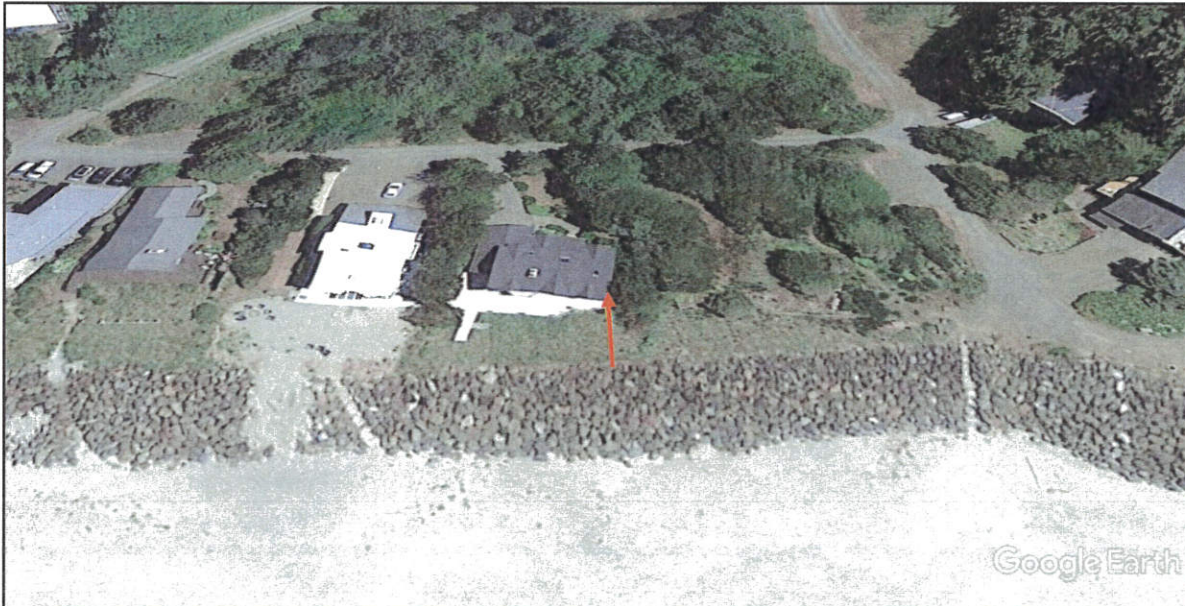
Photo 1 - Oblique east view, Google Earth aerial image dated July 24, 2019.
