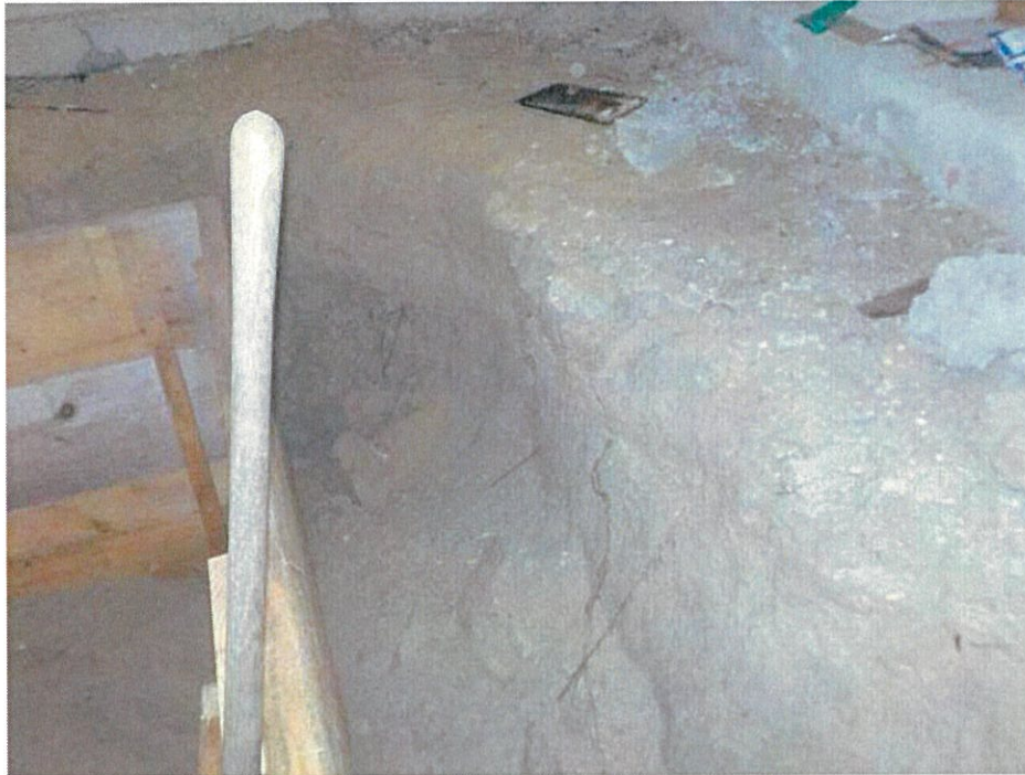
Photo 7 – View of the sand exposed in the crawlspace excavation.
