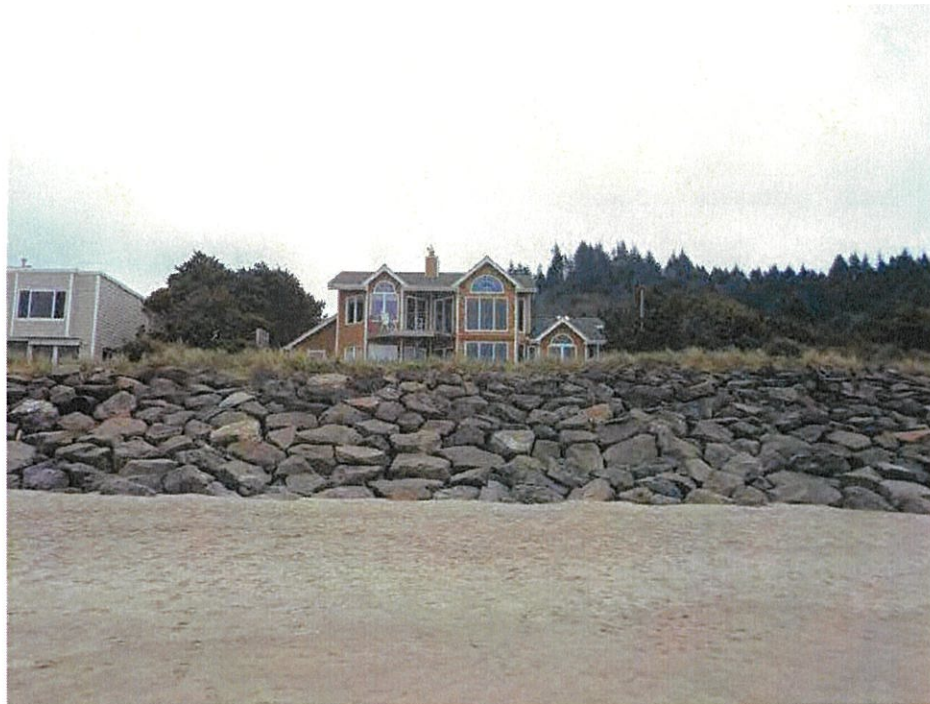
Photo 4 – Easterly view of the site and existing revetment.
