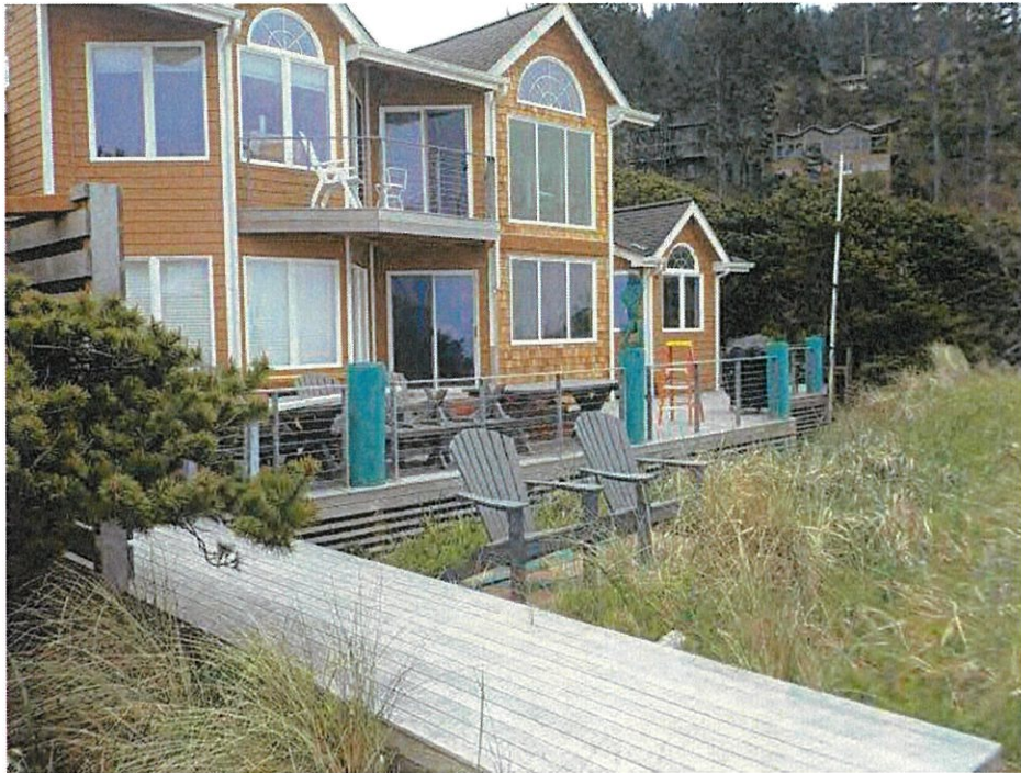
Photo 3 – View of the western side of the existing home and deck.
