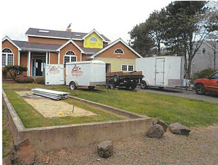
Photo 2 – Northwesterly view of the area of the proposed addition.
