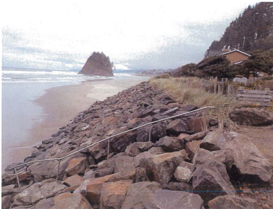
Photo 5 – Northerly view of the revetment, beach access stairs, and Neskowin Beach from just south of the site. Note the continuous riprap revetment along the dune slope.
