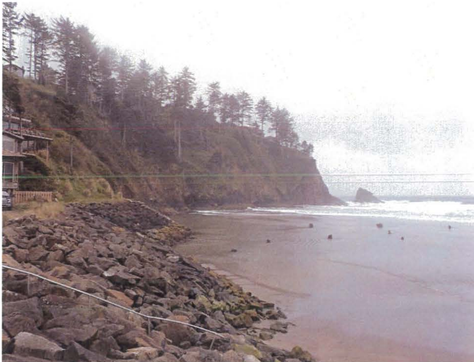
Photo 4 – Southerly view of the beach and bluff from the site. Note the stumps exposed on the beach.
