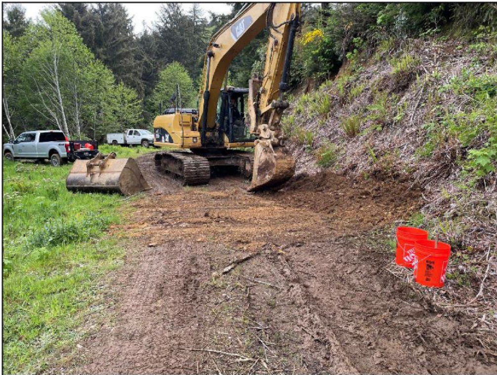
Photo 2: Photo looking northeast along the existing road before the creek. Note that the existing road cut has an oversteepened slope.
