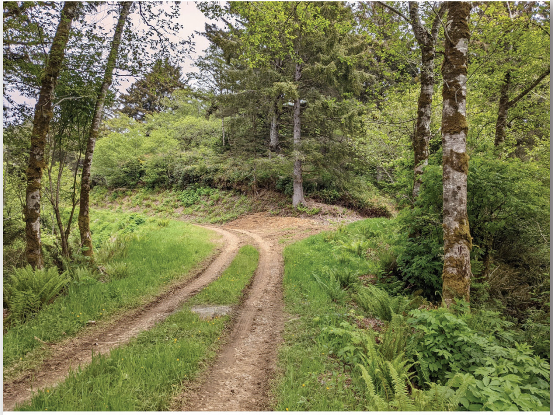
Figure 1. At culvert crossing on Floyd Avenue looking east (P-1)
