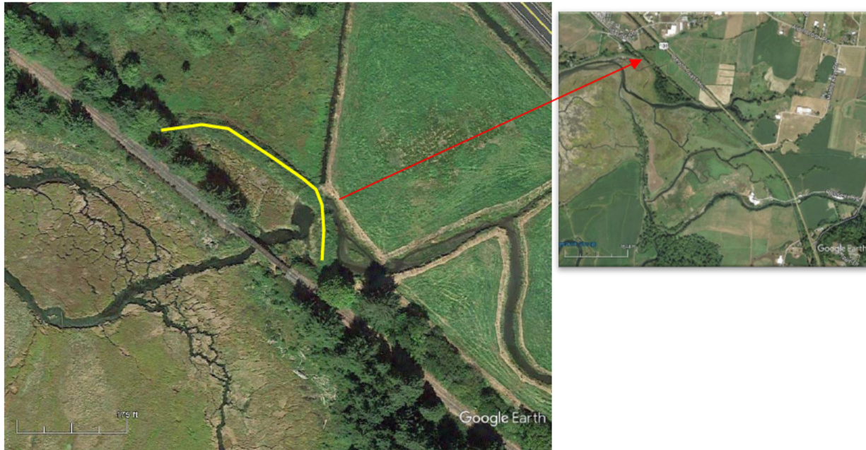
Figure 16: Left - Vaughn Creek Levee - centerline shown in yellow. Right - location on floodplain (August 2016 Google Earth Image)
