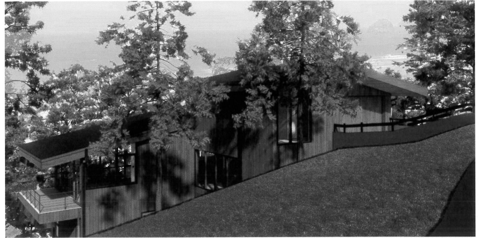
VIEW NORTHWEST FROM NEAR HAYSTACK DRIVE
