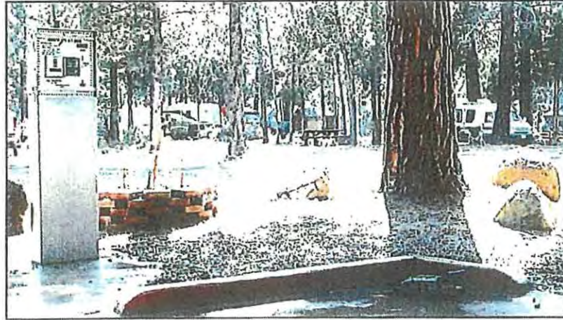
Typical Sanistar paystation location
