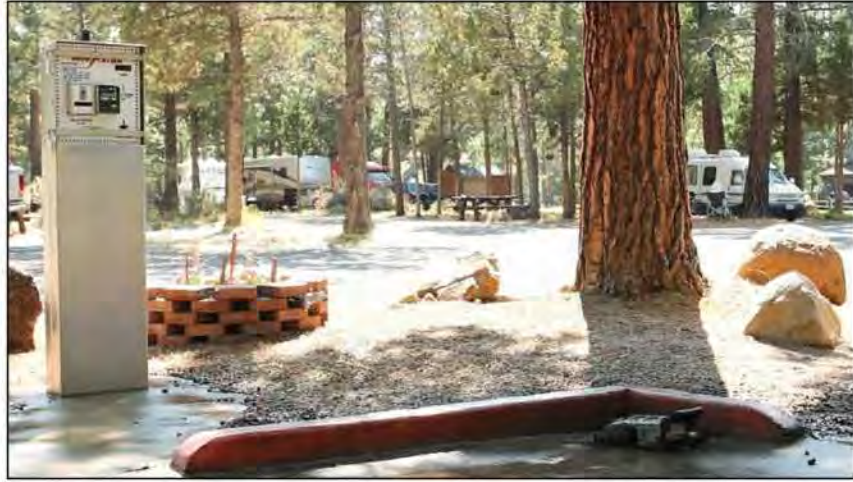
Typical Sanistar paystation location
