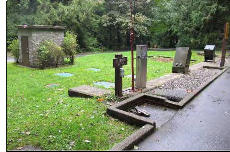
Typical pedestal location
