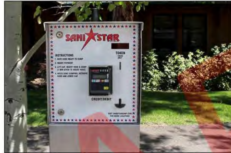
Paystation Close-up. Typical National Rates $10-$25 per dump
