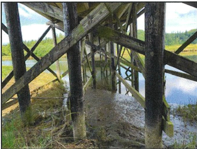
Photo shows the timber trestle substructure extending into the Tillamook River. Here, three piles will be repaired within Bents 6 and 8.
