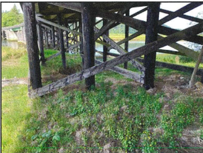
Photo shows the timber trestle substructure from the bridge abutment. Here, three piles will be repaired within Bents 14, 15, & 16. In total, 6 piles will be repaired.
