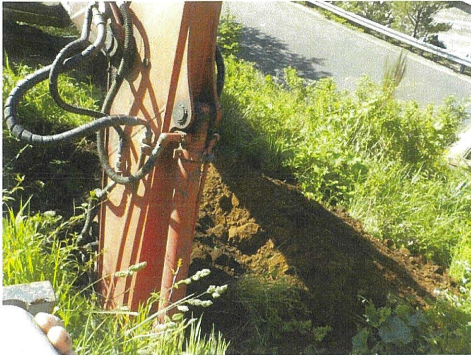
Photo 7 – View of Test Pit 2 being excavated (2018).
