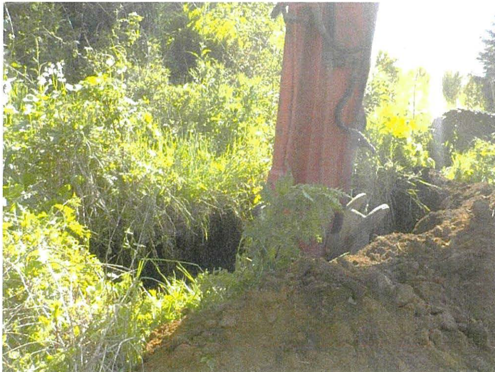
Photo 6 – View of Test Pit 1 being excavated (2018).
