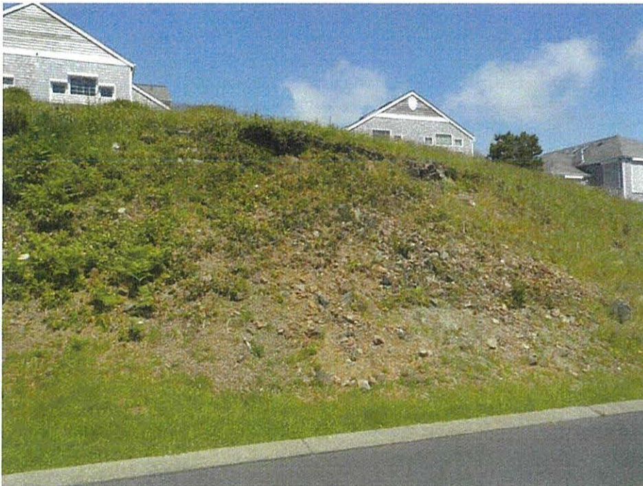
Photo 14 – View of the basalt exposed in a road cut along the north side of Sahhali Drive due north of the site (2018).
