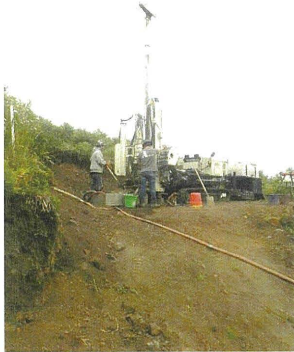
Photo 11 – View of the mud rotary drill rig set up at Boring B-1 (2019).
