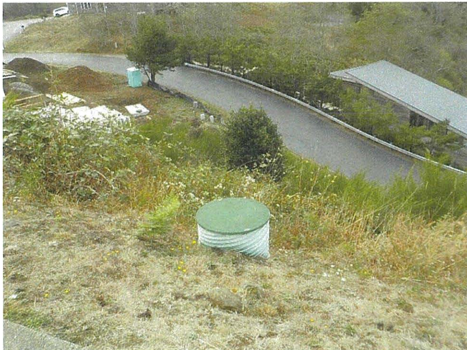
Photo 4 – View of the site from Sahhali Drive looking downslope at the northwestern portion of the site (2022).
