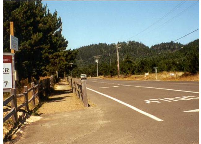
Cape Kiwanda Drive Pathway & Turn-Lane
