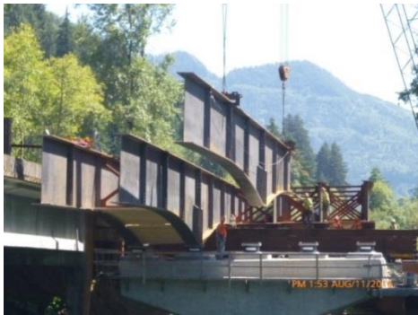
Lommen Bridge reconstruction
