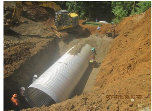
Bixby Road culvert replaced
