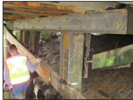
Goodspeed Bridge Repair
