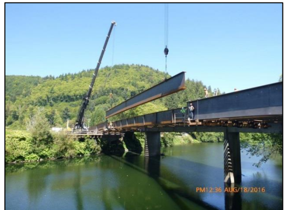
Lommen Bridge Replacement - During
