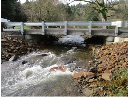
Sifford Bridge replaces a culvert
