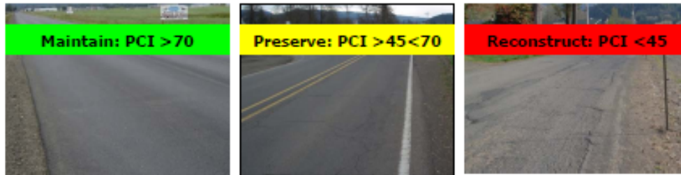
Figure 12 Intervention Strategy & Pavement Condition Index (PCI)
