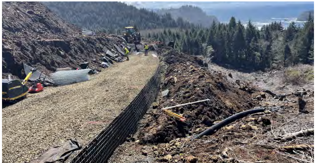
View of MSE Wall No. 2 after the placement of four courses.
