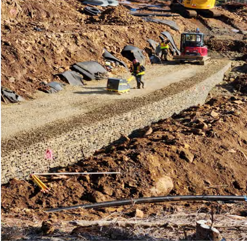
View of completion of the third course of MSE Wall No. 2.
