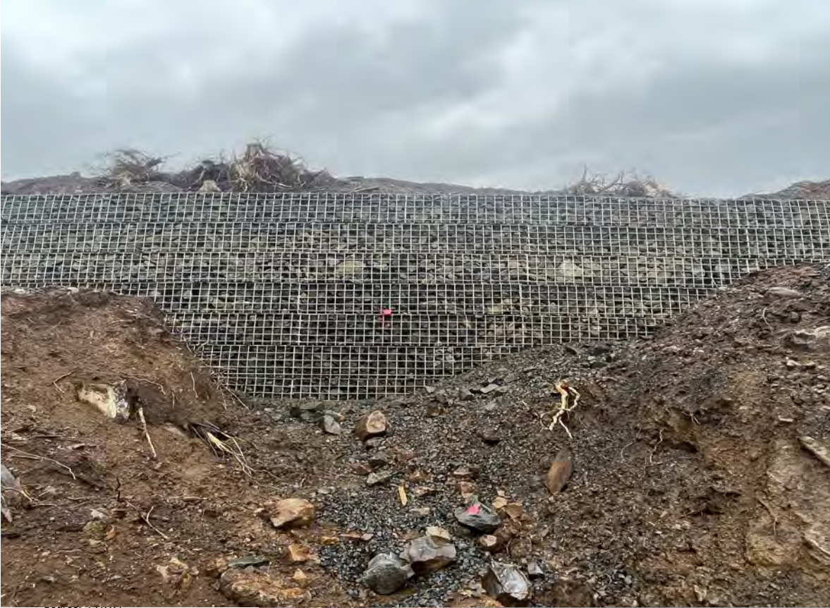
View of face of MSE Wall No. 2.
