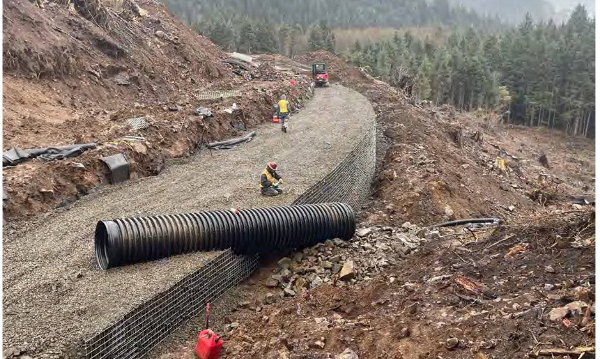
View of MSE Wall No. 2 construction after 7 courses of construction.
