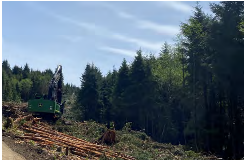
Processing timber on the north side of the project.
