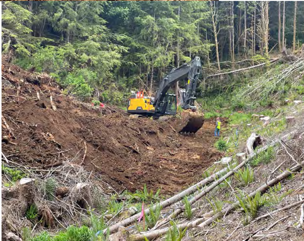
View of 36-inch culvert excavation at Stream No. 2.
