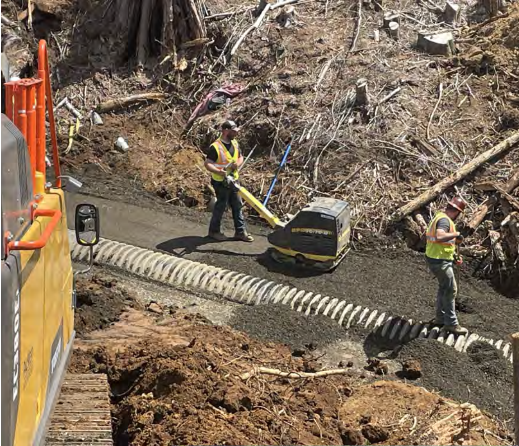
View of backfilling operations for 36-inch culvert at Stream No. 4.
