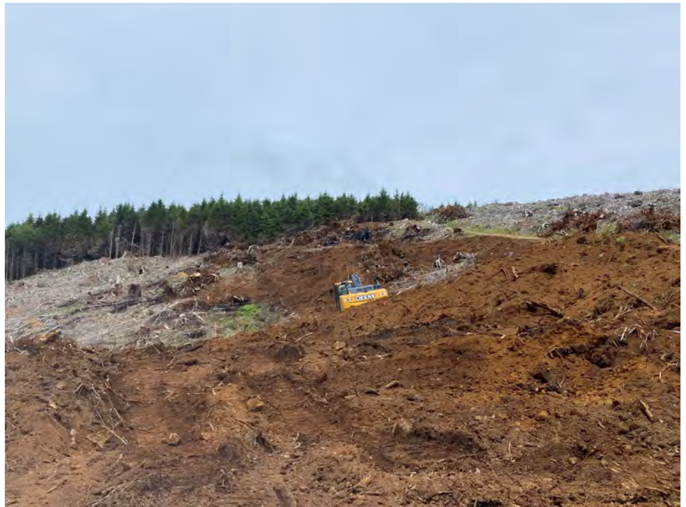
Excavator removing stumps at MSE Wall #3
