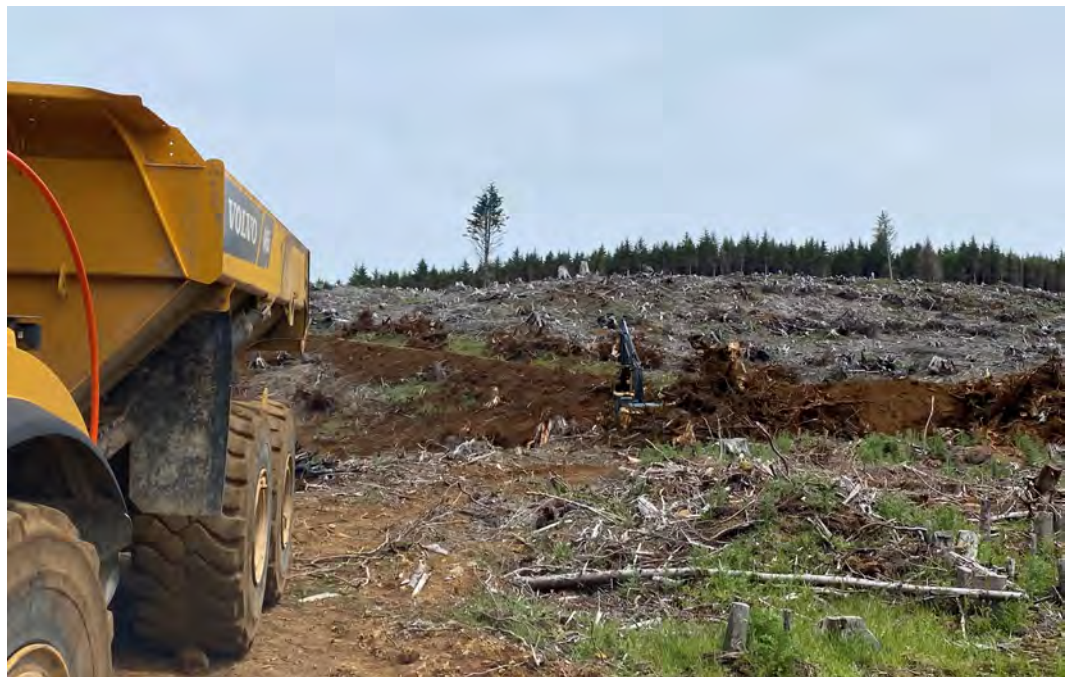
Excavator pulling stumps/ piling slashes
