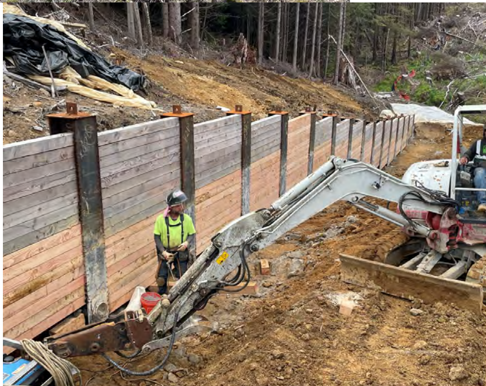
View of soldier pile wall after resuming construction activities.
