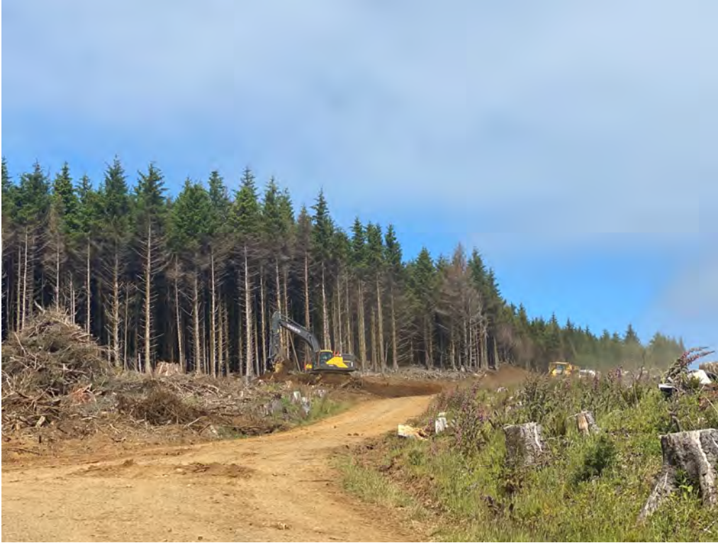
Excavator clearing brushes
