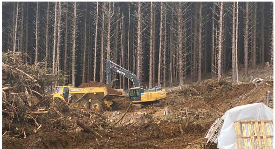
Off road dump truck getting loaded up with topsoil
