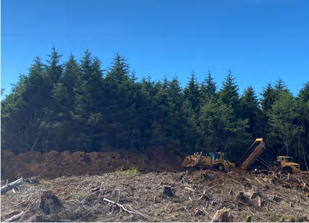
Dozer pushing off conserved material dumped off by the haul truck
