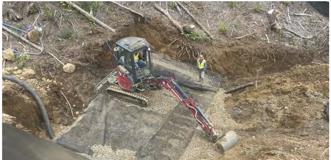
View of bottom course of final MSE wall.
