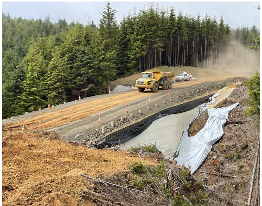
View of hauling operations over the geofoam wall during roadway excation.
