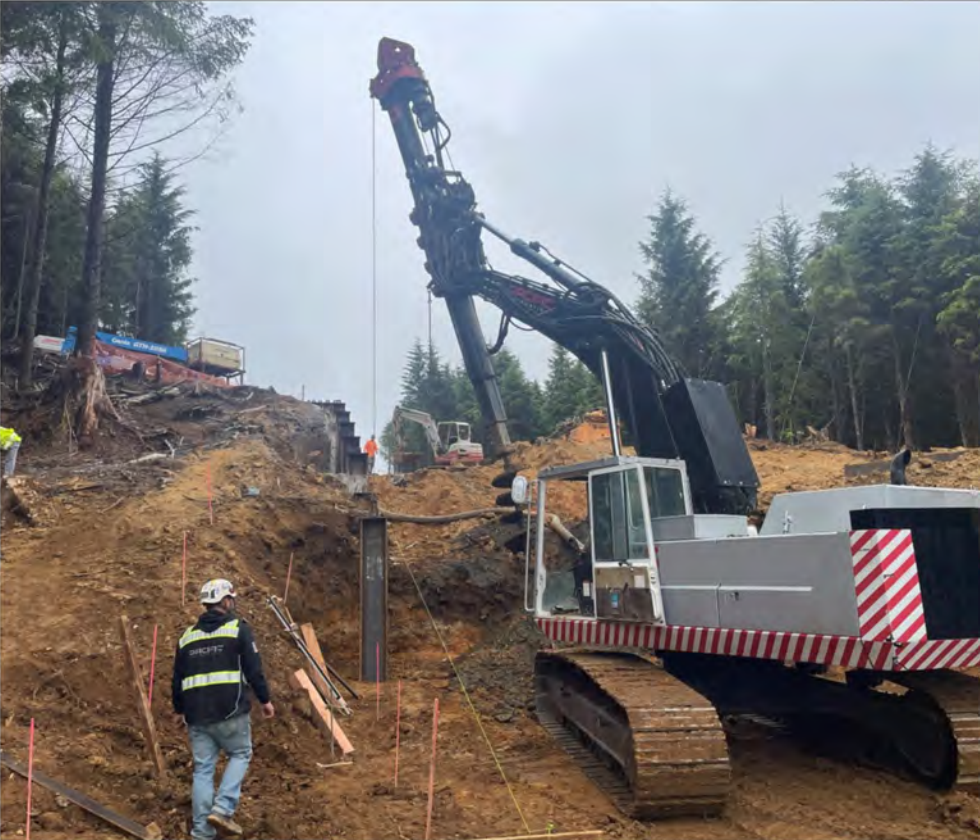
View of pile placement at the soldier pile wall.
