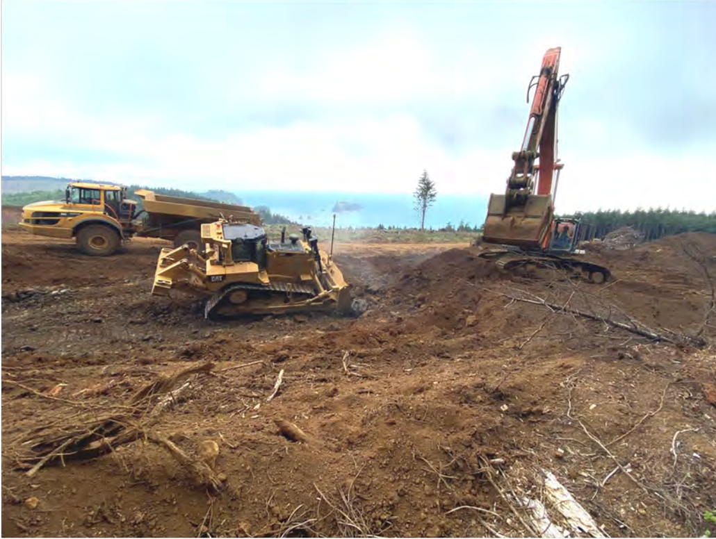
Excavation at st365.
