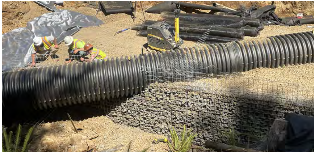
View of MSE Wall No. 1 with culvert after four completed courses.
