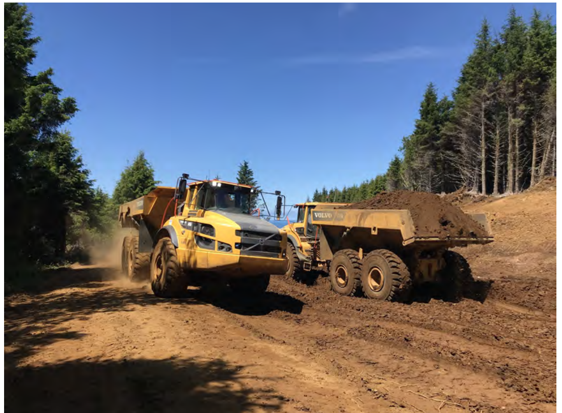
Hauling off exca- vated material
