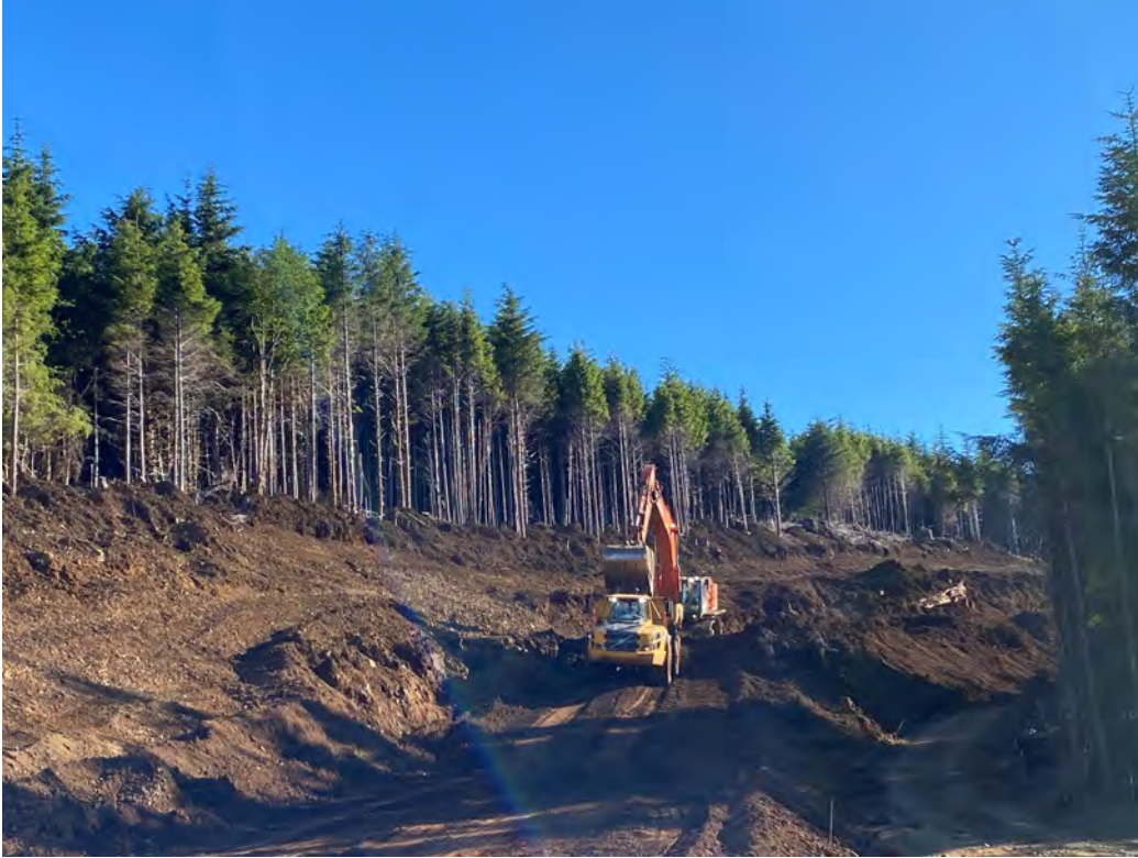
Excavation at st350.
