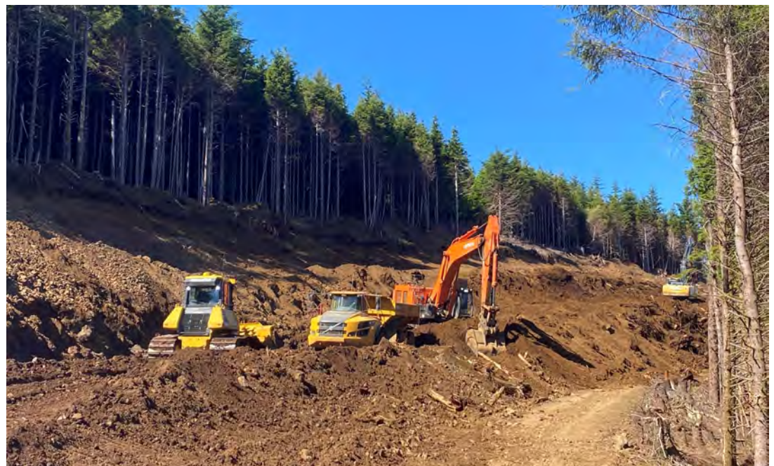
Excavation at st350.
