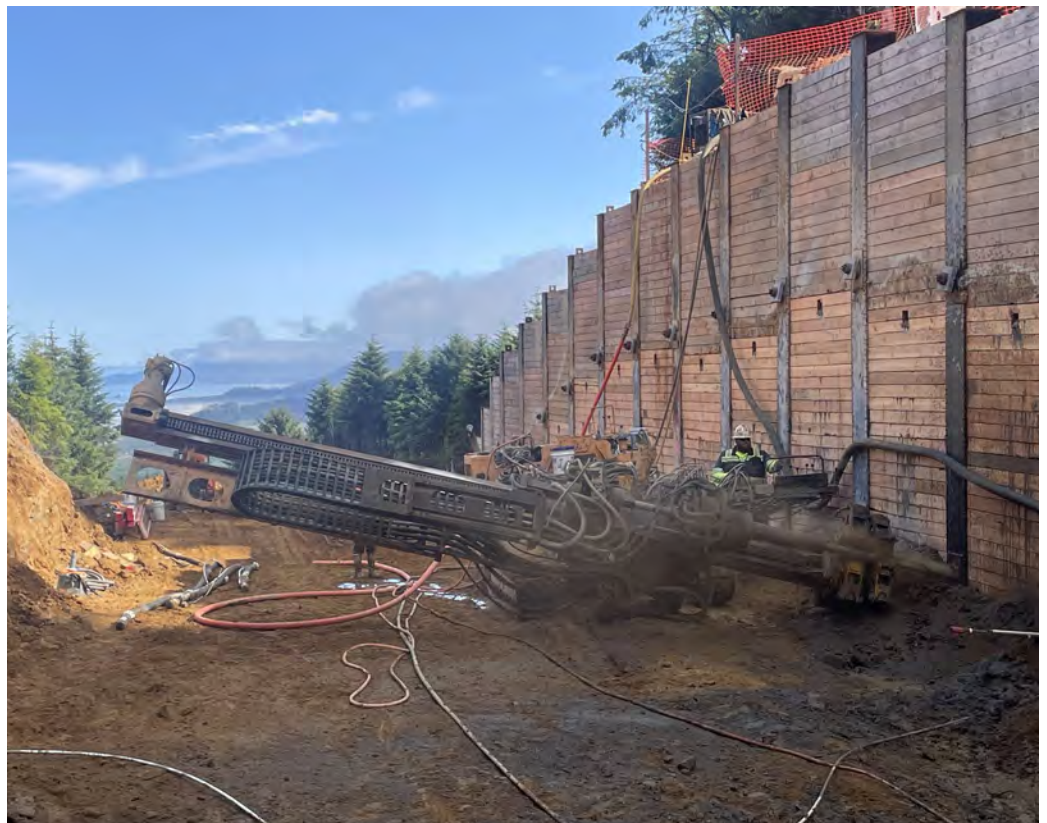
View of ground anchor installation at soldier pile wall.
