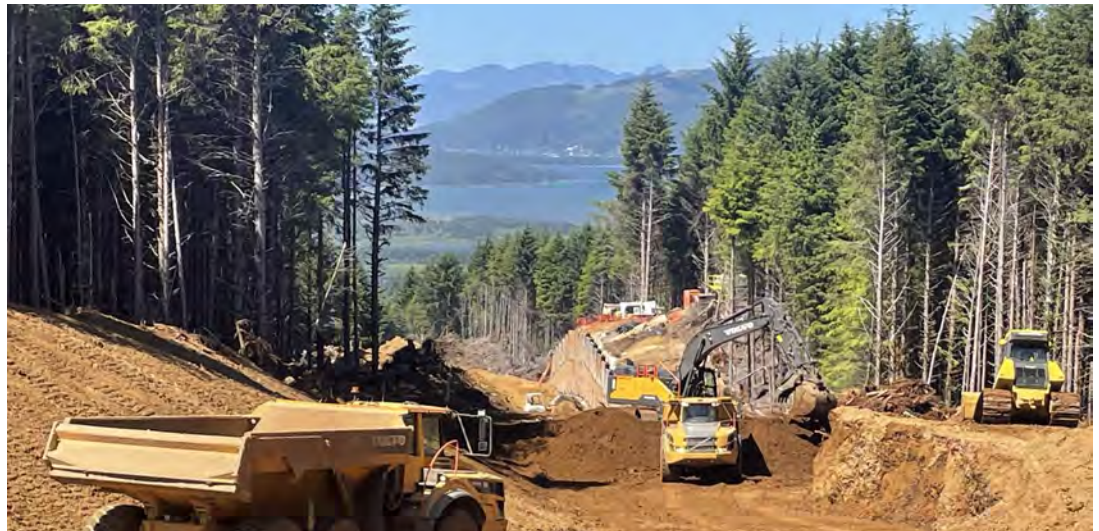
View of roadway excavation showing soldier pile in the background.
