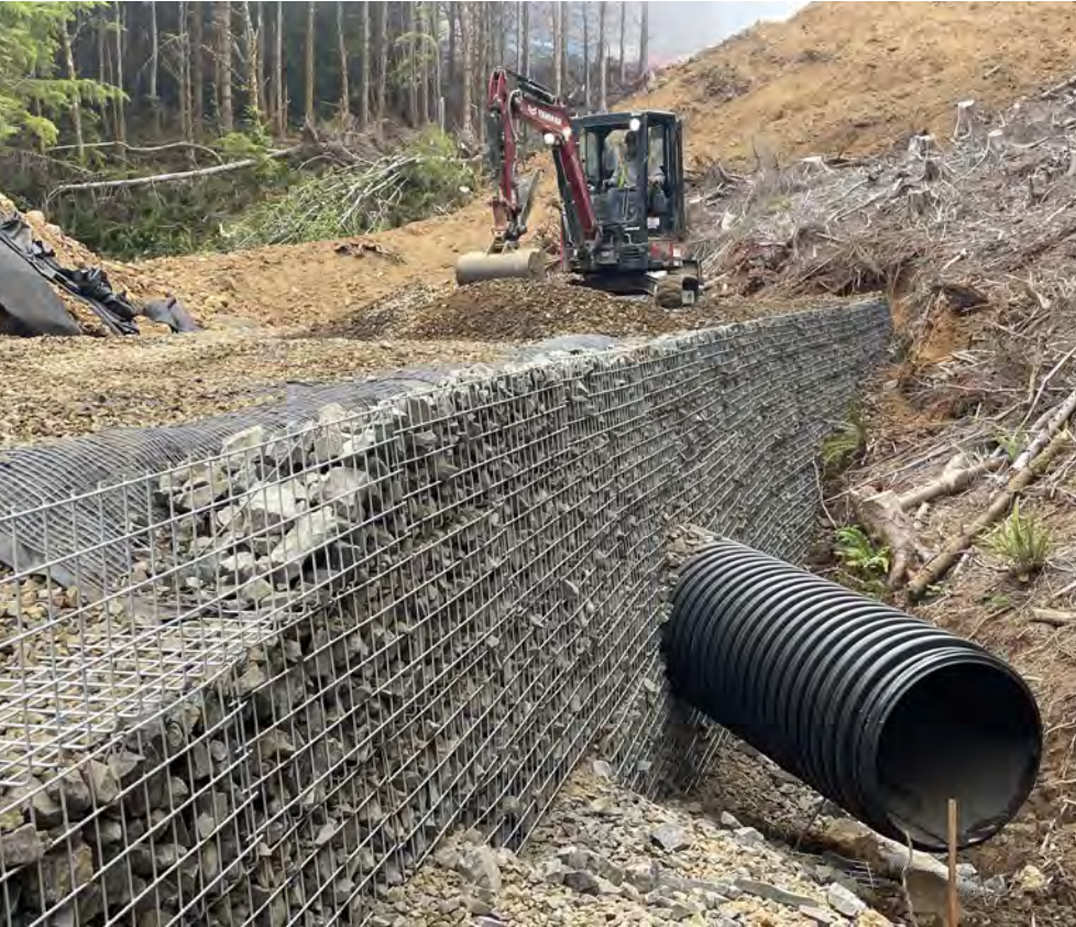
View of MSE Wall construction progress.
