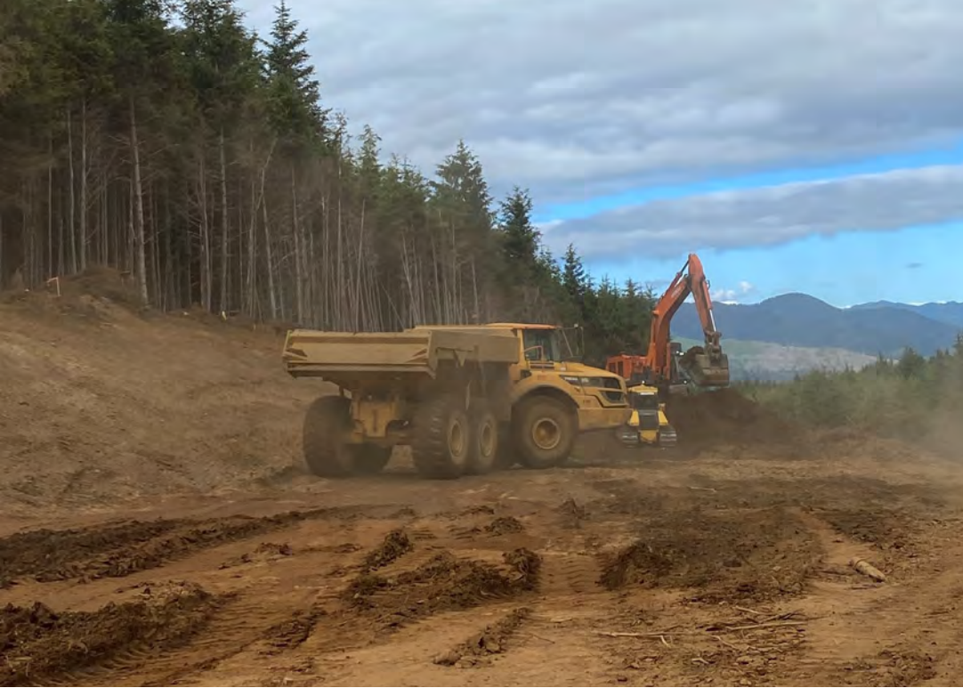
Excavation at st340.
