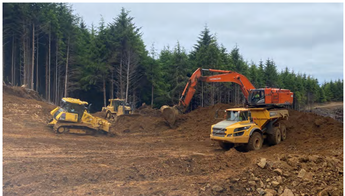
Excavation at st332.
