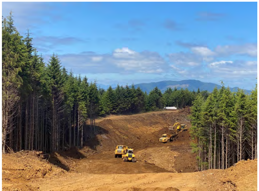
Excavation at st328.
