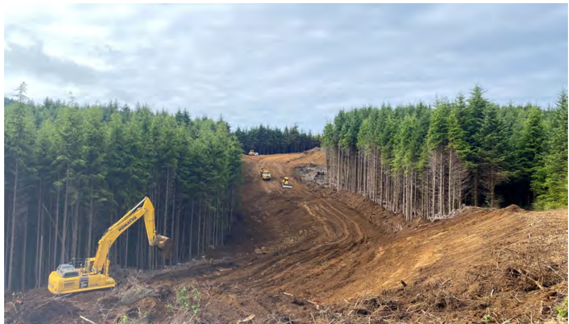
Excavation at st327.
