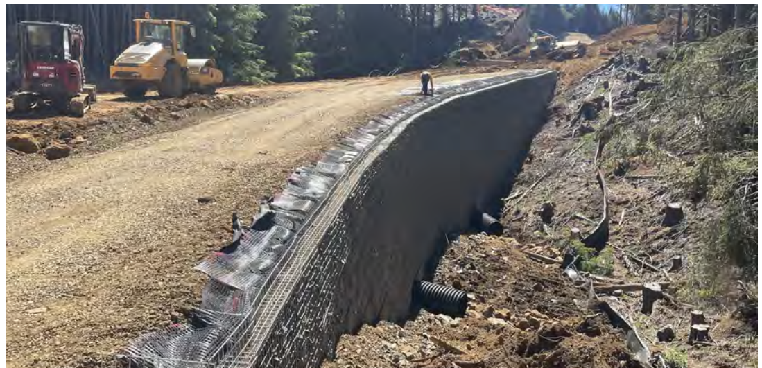
Construction of final course for MSE Wall No. 1.
