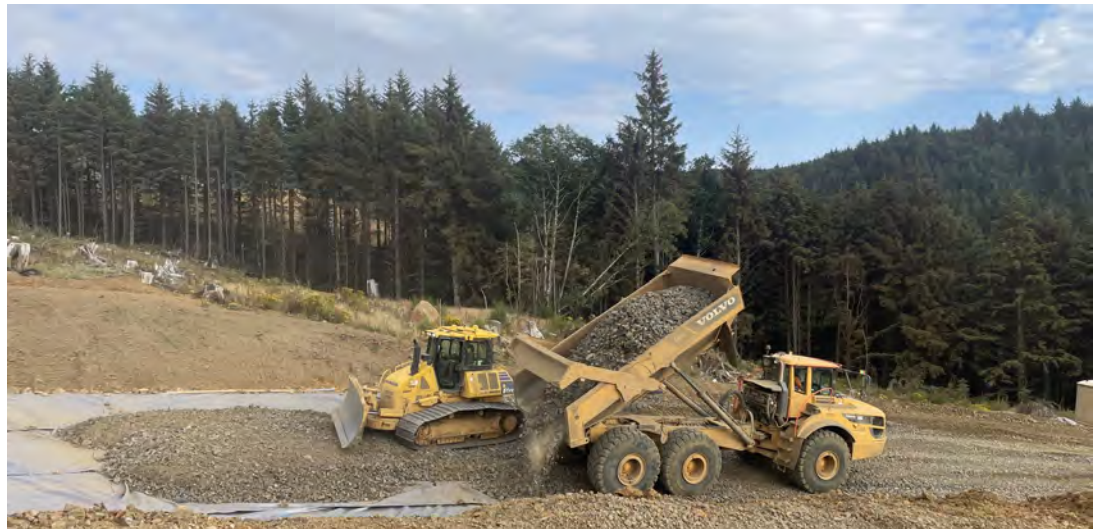
View of roadway aggregate base course placement.
