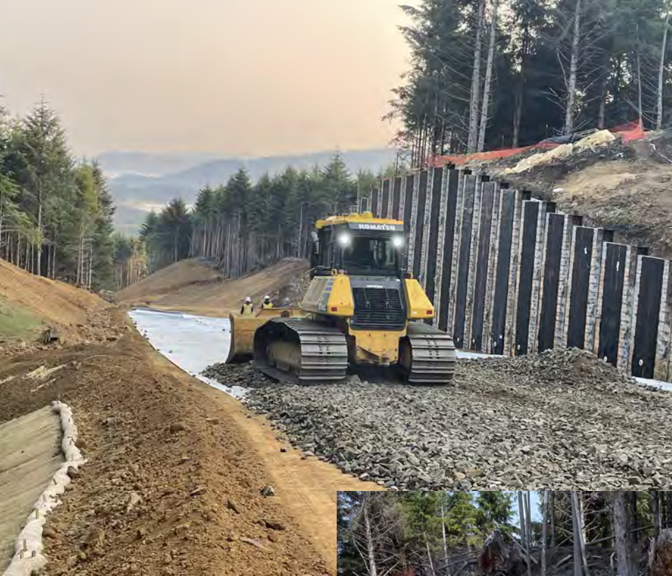
Alternate view of roadway aggregate base course placement.
