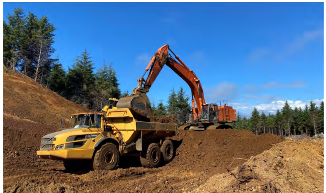
Excavation at st324.
