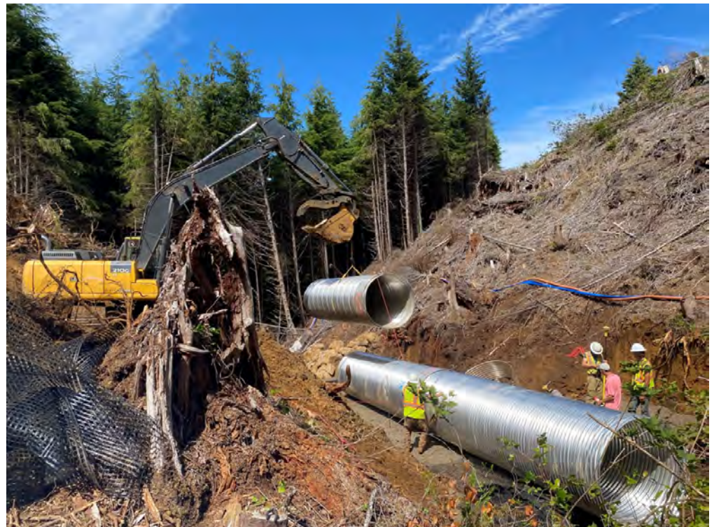
Placing culvert pipe for Coleman Creek
