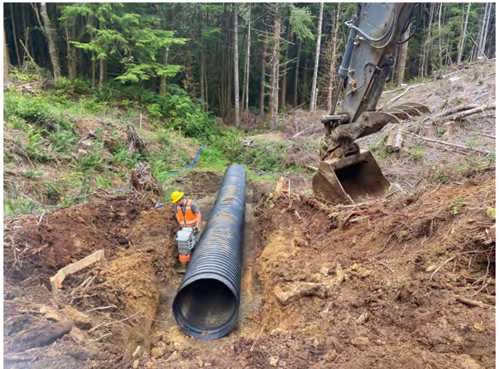
Setting and backfilling the HDPE pipe for Stream 5
