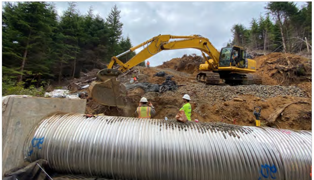
Backfilling the pipe at Coleman Creek.
