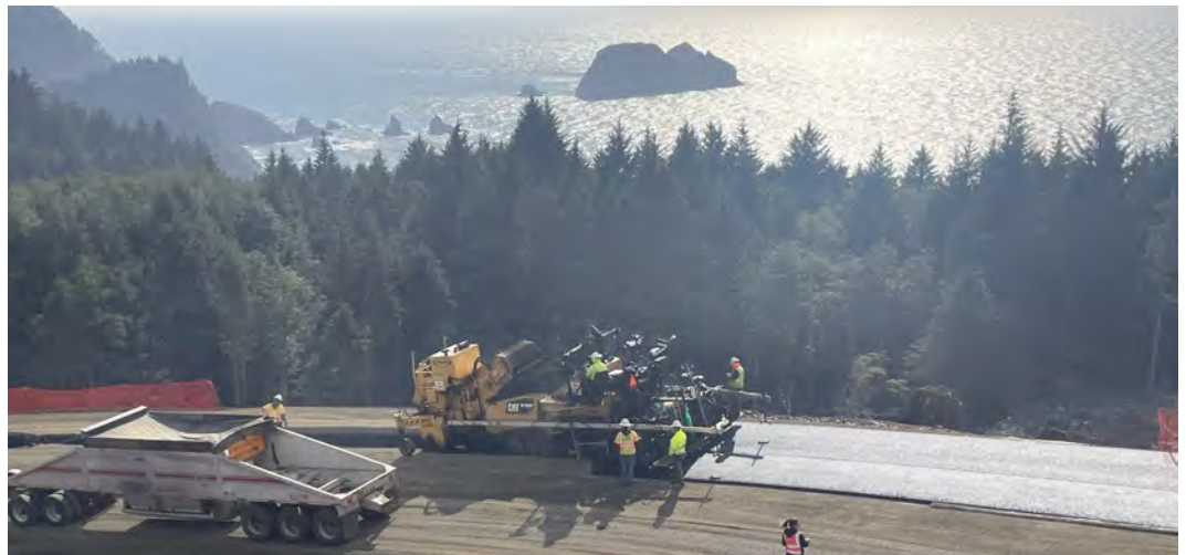
View of asphalt placement overlooking the Three Arch Rocks.
